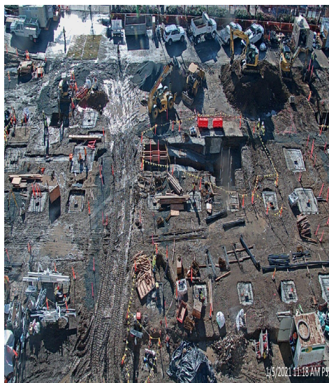
Construction of ZSFG Research and Academic Building, January 2021 Fraser Conrad
