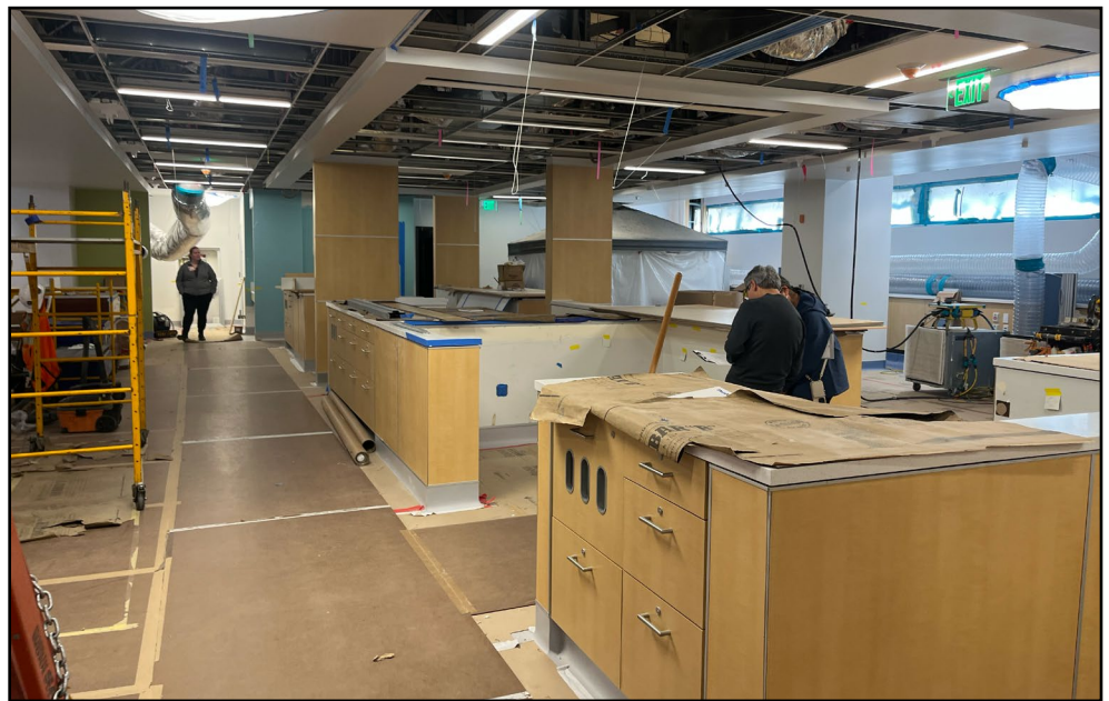
New Outpatient Dialysis Unit Under Construction in Bldg 5, 3rd Floor
